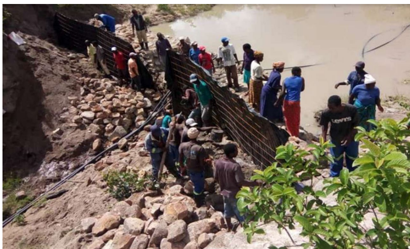
The Manyenga dam, in Mutoko District. Part of the BRAC programme, which is helping communities adapt to climate and socio-economic shocks in Zimbabwe. Photo: Christian Aid
